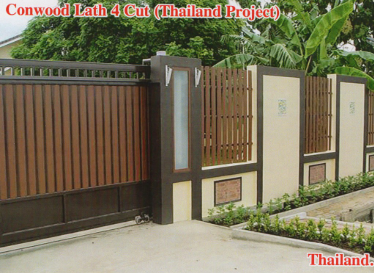
FANCY WOOD FINISH GATE PLEASANTS THE ENTRANCE
